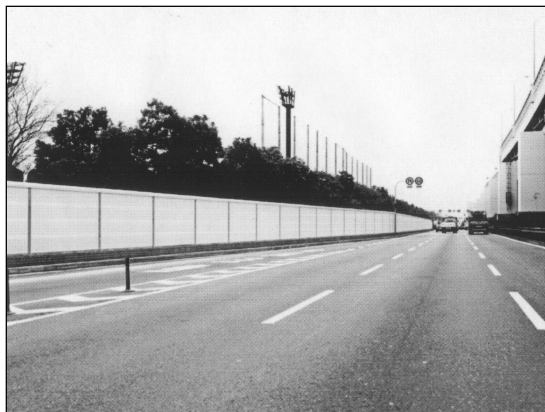
Fig. 5 View of soundproof highway walls coated with titanium oxide photocatalysts for the elimination of NO x . These new walls were constructed in Osaka, April 1999.
